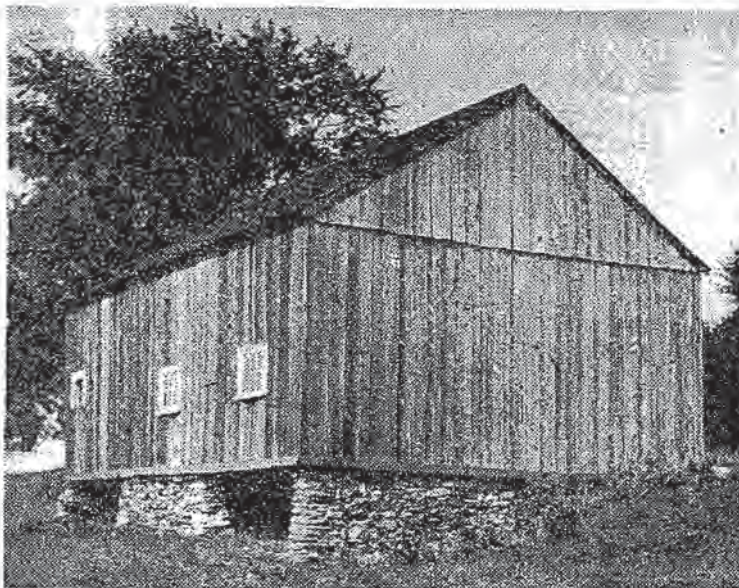
The old horse barn at Marlboro, Vt., as it looked before the students and faculty members went to work making changes.
