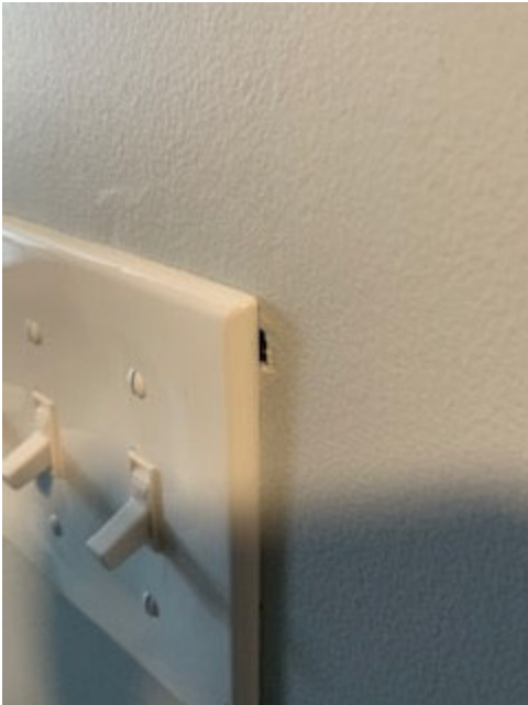
holes cut incorrectly for light switch receptacles
